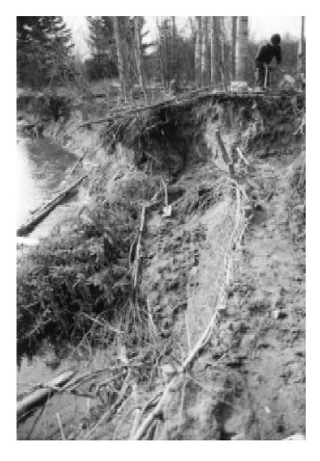
vent undermining at the upstream end of the main structure since it was expected that the upstream end of the spiling would bear the brunt of increased water current. Two small spruce tree revetments, anchored by 1/4" cable to a nearby cottonwood, were woven into this short section of spiling (Photo 2).
