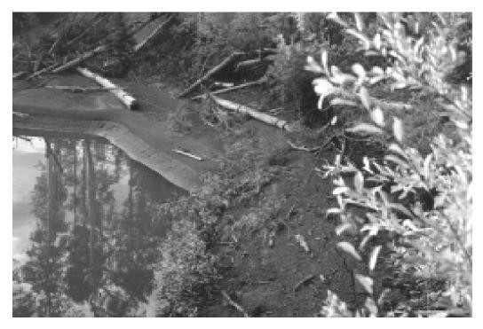
devoid of needles. The contour wattling showed signs of degradation as wattles were becoming exposed. This suggests that the wattles were not sufficiently buried when initially placed or that they had become exposed by erosion. The short sections of wattling covered by contour wattling, one wattle long by three wattles high, may also have adversely affected this section's stability. Longer sections of contour wattling may be less prone to exposure or downslope move-
